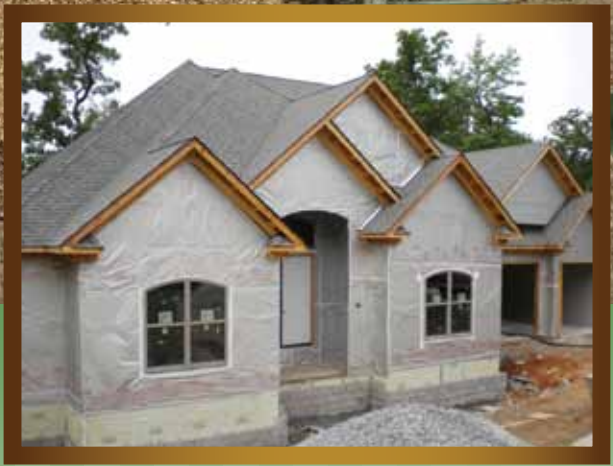
Home wrapped and flashed with DuPont Tyvek ThermoWrap.
