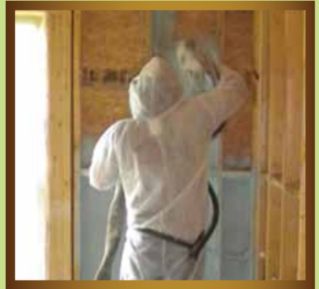
Closed cell foam insulation being applied.
